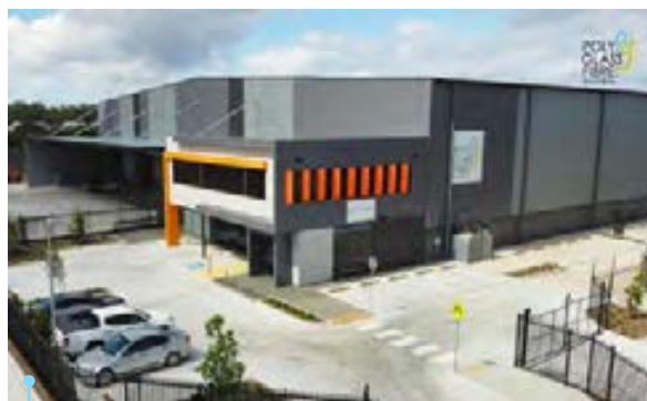
Brisbane, Queensland Operational since May 2023
