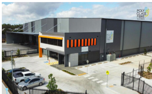
Brisbane, Queensland Operational since May 2023
