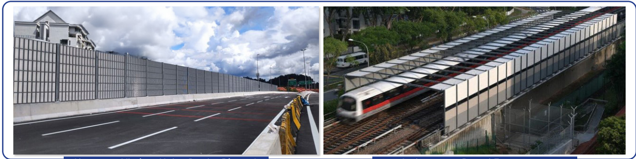
Singapore Viaduct Noise Barrier Phase 2.
