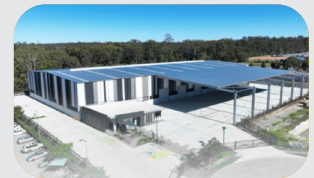
PGF Insulation Pty Ltd Heathwood, Queensland 6,019 sqm warehouse + 312 sqm office
